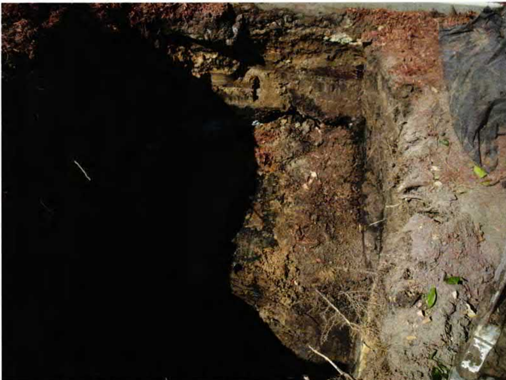
Picture 2: UST 308Ash excavation in progress.
